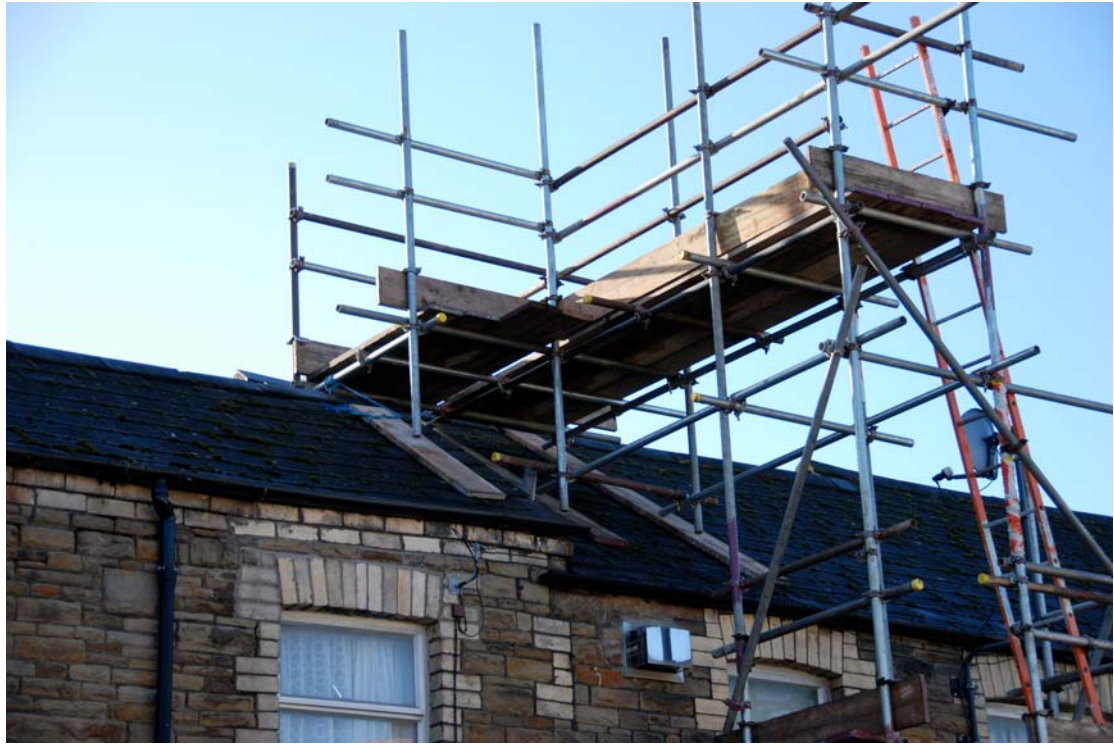
Figure 5: Scaffolding extending over ridge
