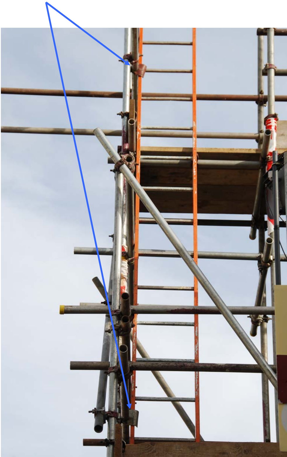
Photograph by Richard Neale Figure 4: Detail of ladder fixings
